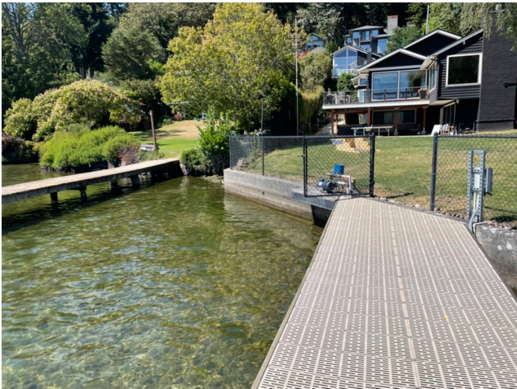
Photo 4 - Existing shoreline conditions looking south.
