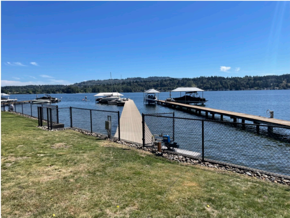
Photo 1 - Existing dock looking waterward.
